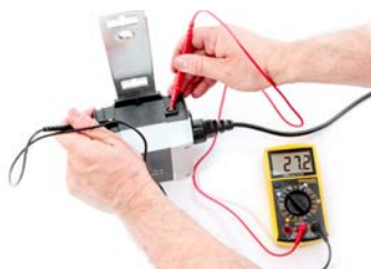
Checking voltage on charger
